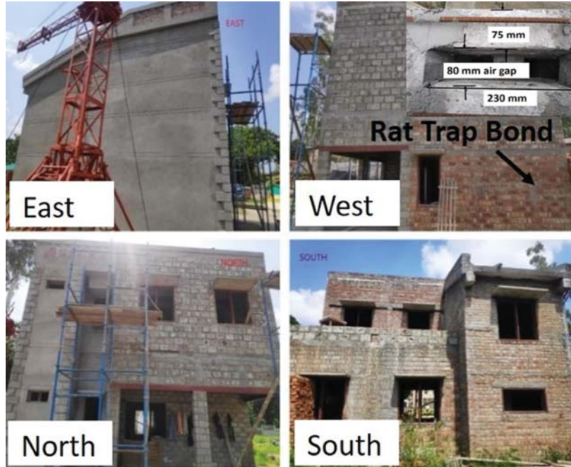
Fig. 5. Directional faces of brick wallbuilding.
