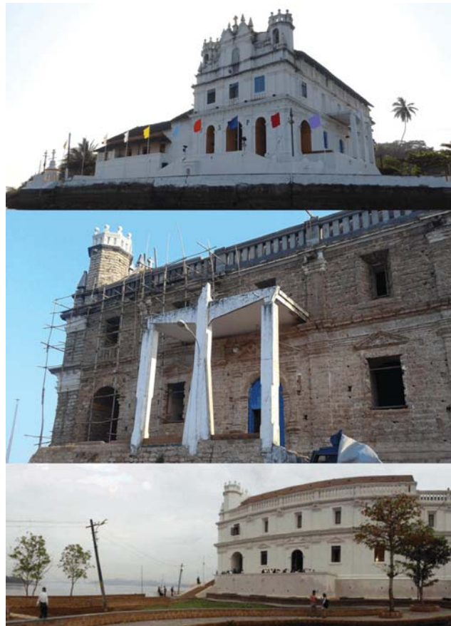
Fig. 6. Nossa Senhora de Penha de França church, Goa - India (pre- and post-restoration).
